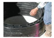
3. Now that you have your preliminary measurements, you will need to determine the best ring height combination to attain the necessary adjustment for your specific installation. In cases where grades are not flat, use slope rings to accommodate for this difference.
