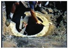
1. The first step is to make sure you have a clean installation area. Be sure to clean the concrete cone or top slab with a whisk broom or chisel. This will assure a flat seating surface free of rocks, gravel, blacktop, protruding concrete or frozen debris.
