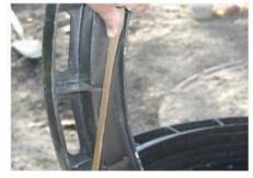
**8.** As before, place the second ring down onto the first with the male lip interlocking into the center of the first ring. For each ring, make sure to line up your paint
