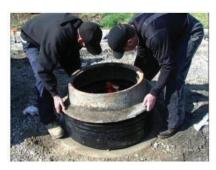
11. You will now proceed to install the cover frame. Prior to setting it in place, apply a 3/16-to-1/4-inch bead of the approved caulk butyl sealant or a minimum of 3/8 inch round rope ASTM C-990 on the top of the last ring. Be sure to apply the sealant in a location so that it contacts the cover frame the full 360 degrees. If necessary, you may apply a double bead of sealant.
