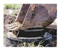
**13.** At this point, the installation of your LADTECH adjustment rings is almost complete. The final step is to press down with a back hoe bucket compressing the butyl rubber between all the rings.
