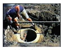
2. With the installation area now clean, measure the distance from the cone or top slab to the projected finish grade. When making this measurement, be sure to deduct the distance, or height, of the cover frame. Determine the net build-up of rings necessary to achieve final the grade with the cover frame in place.
