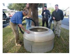
1. The first step is to make sure you have a clean installation area. Be sure to clean the fiberglass cone with a whisk broom or glove. This will assure a flat seating surface free of rocks, gravel, blacktop, protruding concrete or debris.
