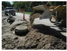
**13 a.** As you can see you can immediately backfill or concrete encase the installation area and proceed to your next installation site.
