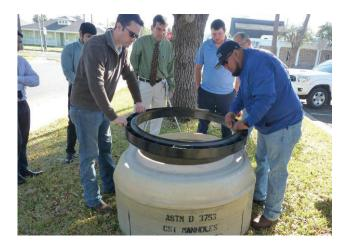
7. With the sealant applied, place the first ring down onto the cone or top slab with the male aligning lip facing up. Make sure to line up your paint strip.
