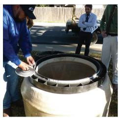
**8.** As before, place the second ring down onto the first with the male lip interlocking into the center of the first ring. For each ring, make sure to line up your paint strip.
