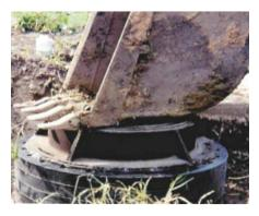
**12.** It is important now to compress the butyl mastic sealant completely. This can be accomplished by having several people stand on the final installation and walk around, or by having a backhoe knuckle down on the top of the ring and cover
