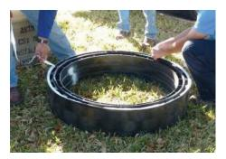
**6.** You are now ready to begin the actual installation. With all rings within arm's reach, apply a minimum of 3/8 inch round butyl rope ASTM C-990 to the flat surface of the rings facing up. Be sure to apply a second rope on the outside to ensure a complete seal. Be sure to cut the butyl ¼ inch long with a knife or sharp instrument and knead the two ends together so the splice cannot be seen.
