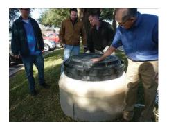
**4.** With the measurements determined and your required rings selected, dry stack the rings on the cone or top slab. Rotate any slope rings as necessary. With the rings dry-stacked, place the cover frame casting on top of the assembly and verify the height and slope match.
