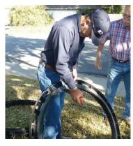
**9.** for the final top ring only, snap off the aligning lip using flat nose pliers and rocking the lip back and forth until it snaps. Continue around the entire ring until the entire aligning lip is removed. This ensures a flat sealing area for the frame and cover.
