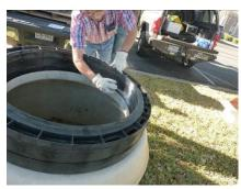
**5.** When the assembly is in place and you have your desired height and slope, mark the entire stack and manhole cone with a vertical line of spray-paint. Once you have your line, remove the entire stack as one unit and place upside-down on the ground next to the manhole.
