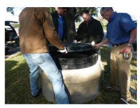
11. Gently place the frame and cover onto the final ring, being careful to ensure it is centered prior to placing it on the Ladtech rings and Butyl mastic sealant. DO NOT KICK OR DROP FRAME AND COVER INTO PLACE as this will result in an improper installation that will have to be completely disassembled and reassembled from the top of the fiberglass cone up.
