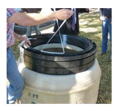
**10.** At this point, apply 2 separate rings of butyl mastic to the top ring to ensure a tight seal with the ring and cover. Make sure the 2 rings of sealant are side by side, not on top of each other.
